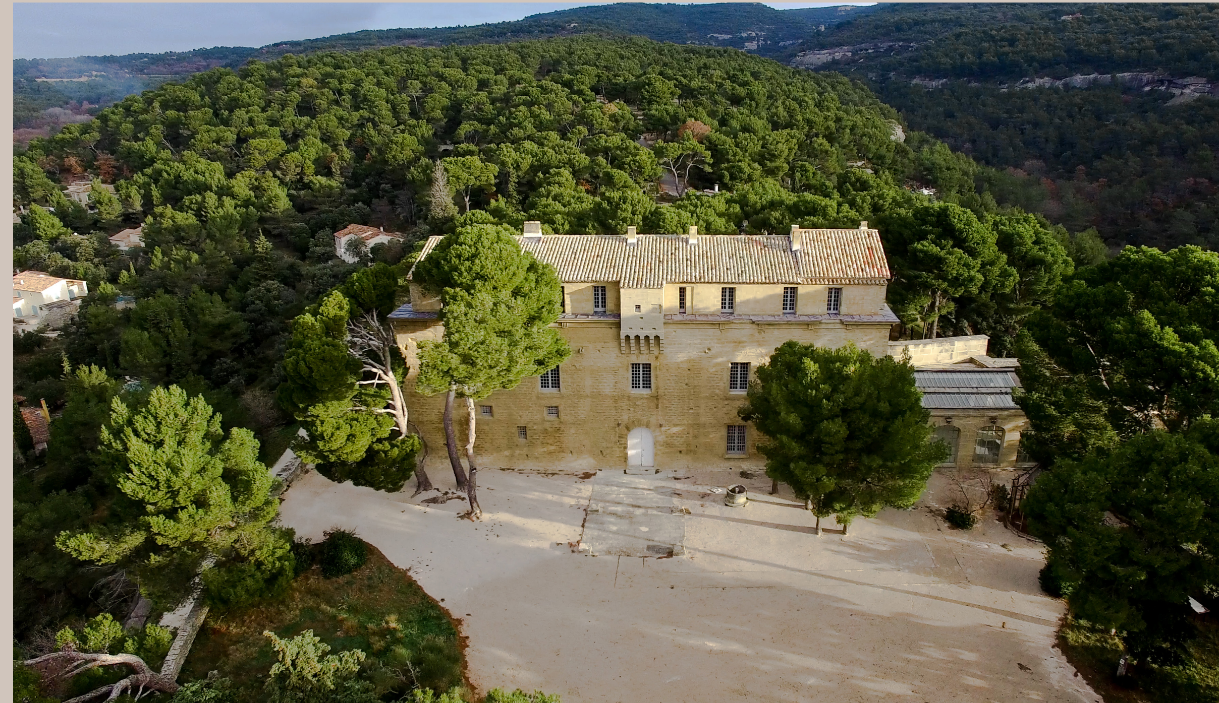
South façade : the medieval main house, the orangerie and the esplanade
