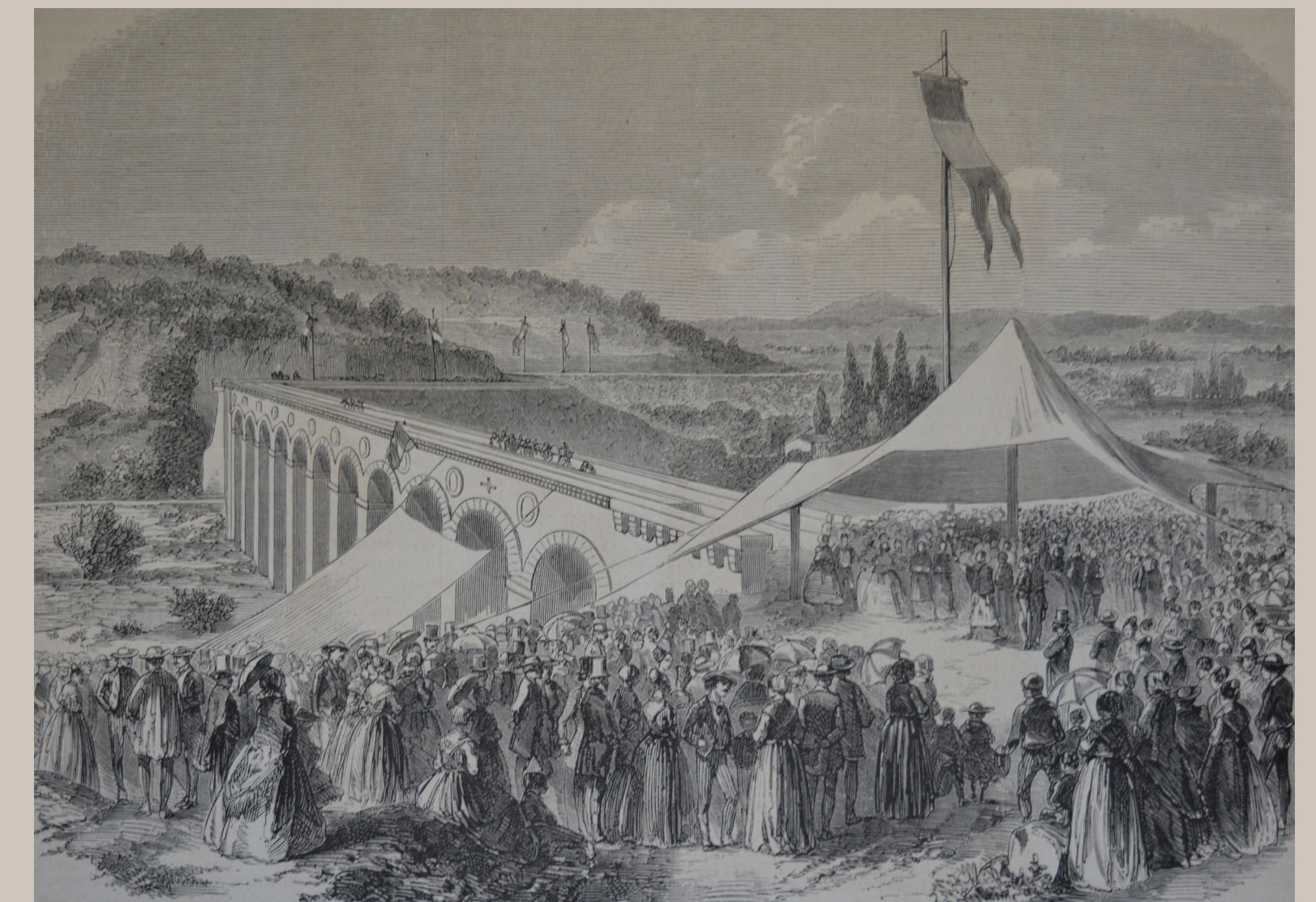
The inauguration of the Galas aqueduct in the presence of Empress Eugénie. Drawing by J.B. Laurens in the L'illustration magazine, dated 25 July 1857 © Bibliothèque-musée Inguimbertaine, Carpentras
